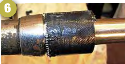
6 Use good quality tape for protection
